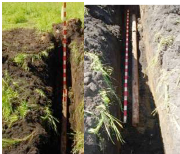
Fig. 14. Steel pipe with length of 4 m, D=100 mm. Deployment depth is 1 m.
