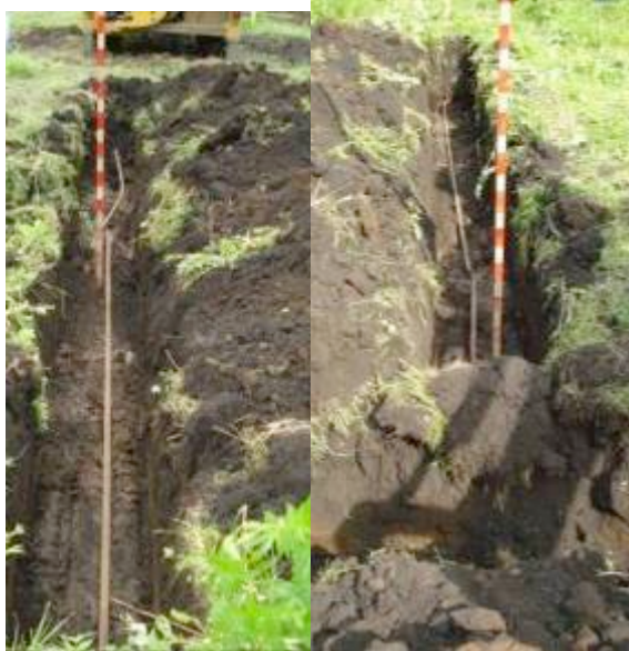
Fig. 33. Iron bar with length of 7.5 m. Cross-section 20*30 mm. Deployment depth is 0.7 m.
