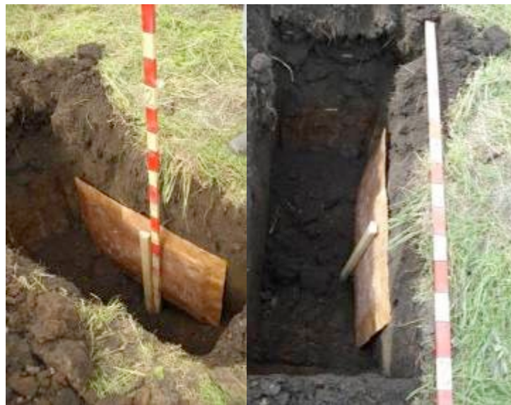
Fig. 28. Vertical copper sheet 1*0.6 m. Depth down to the upper face is 0.45 m (Put on the 1m side).
