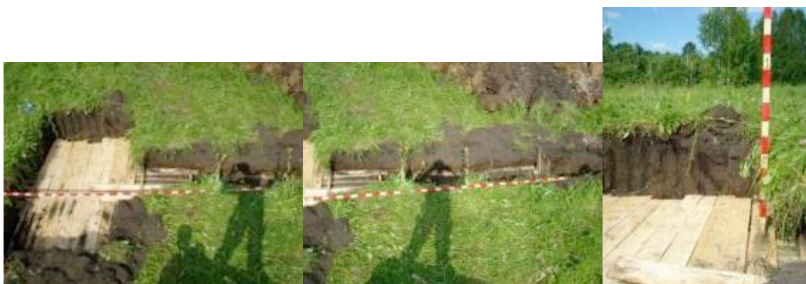
Fig. 16. Dig-out (room 2*2 m and corridor 1*3m), the roof is at the depth 1 m, the dig-out depth is 1.5 m.
