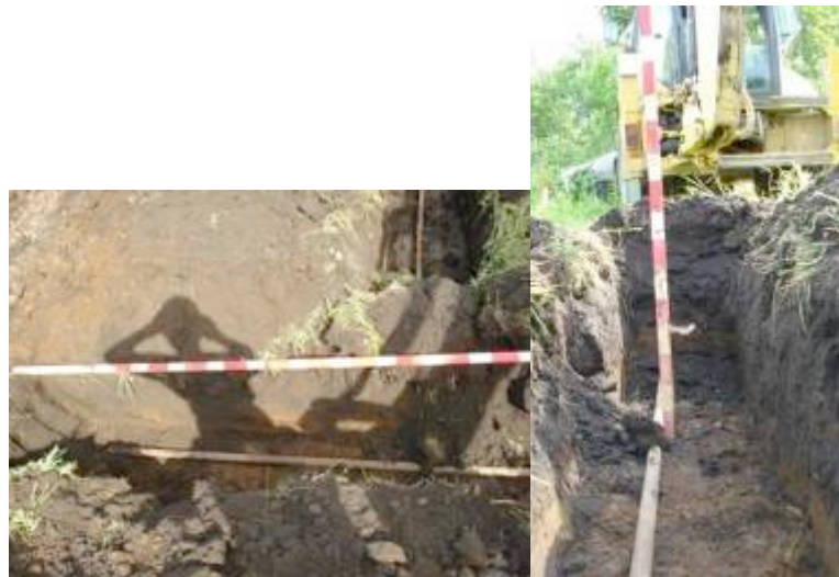
Fig. 32. Steel pipe with length of 3 m, D\ 42 mm. Deployment depth is 0.65 m.
